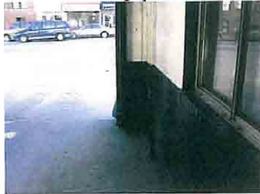
Fill Line Parking Garage 4650 Broadway, New York, NY
