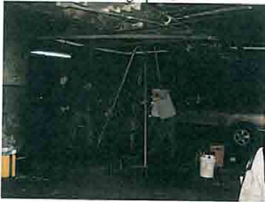
Soil Boring SB-01 in Progress 4630 Broadway, New York, NY
