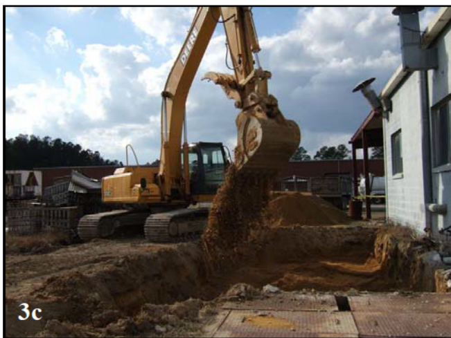
Figure 3: Photo Documentation of a RegenOx Excavation Application.
