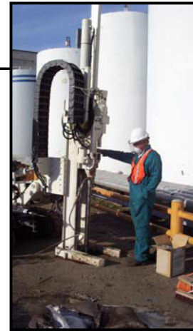
Figure 1. On-Site Direct Push Injection
