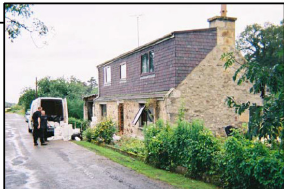
Figure 1. Cottage with fuel oil spill
